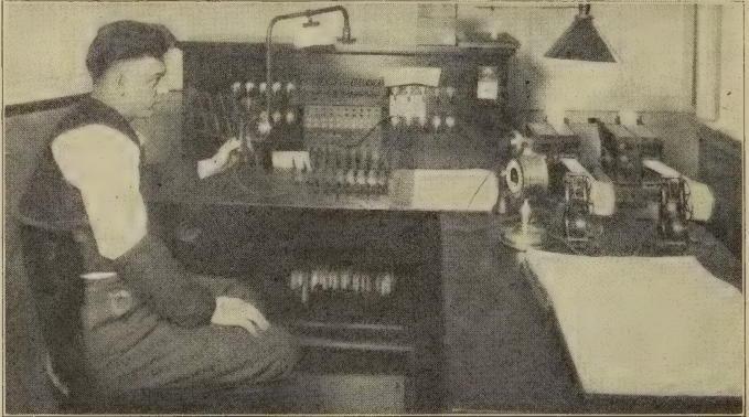
SWITCHBOARD IN POLICE DEPARTMENT OF DAYTON, OHIO
